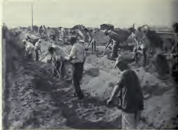
project near Salerno. The rock base is 20–25 centimeters thick. Each man working on the irrigation canal for this project moves on average of 4 cubic meters of earth each day—see photo above.
